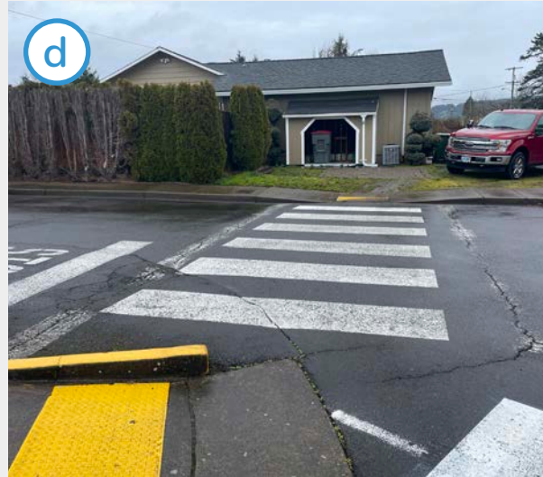
Curb ramps with yellow tactile warning surfaces (in compliance with the ADA) are present at the intersection of Cornwall St and 3rd St, but concrete curbs hinder a smooth transition from roadway to sidewalk.
