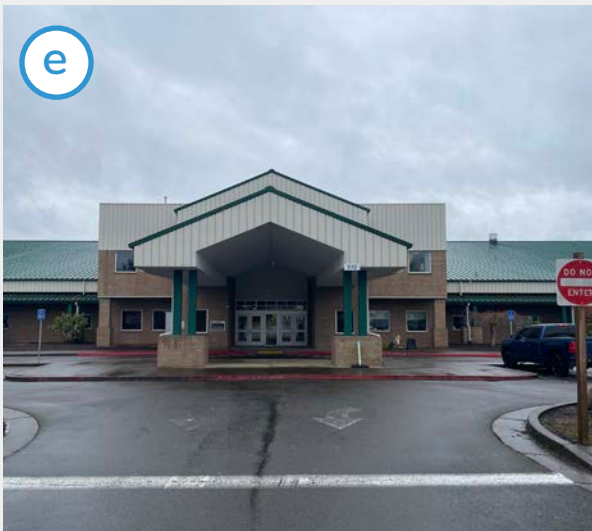
The front entrance to Faulconer-Chapman is covered. Unlike 2nd St and 4th St, there is no continuous sidewalk connecting the entrance to 3rd St; people must cross the bus lane and parking lot to walk on 3rd St.
