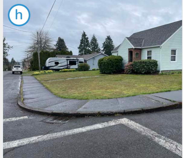
The curbs at the corners at Jefferson St and 3rd St are not ADA compliant.
