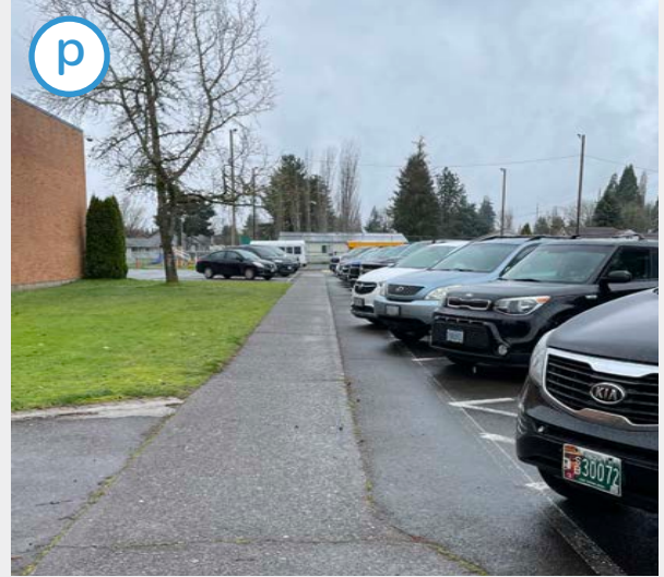
Most stalls in the high school parking lot lack concrete curbs to prevent encroaching into the pedestrian space.
