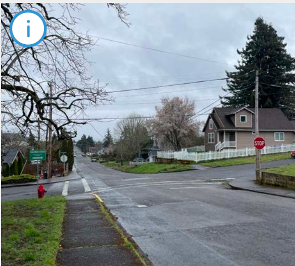
The crosswalks at the intersection of Jefferson St and 2nd St do not use continental markings. The southeast corner of the intersection is a staircase rather than a curb ramp due to the hill.
