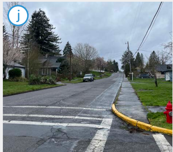
ADA-compliant curb ramps are also missing on the north leg of the intersection of Jefferson St and 1st St. However, the curb ramps on the south leg of the intersection are up to date.
