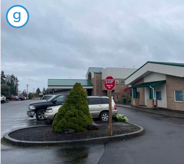
While helpful for managing traffic, this stop sign is not mounted at the correct height.
