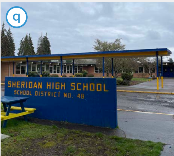
The west side of the high school has a covered walkway where students can be picked up and dropped off.
