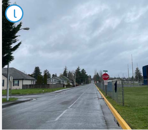
East of Bridge Street on Jefferson St, sidewalk is only present on the southern side of the roadway. The north side of the roadway is immediately adjacent to the high school track.
