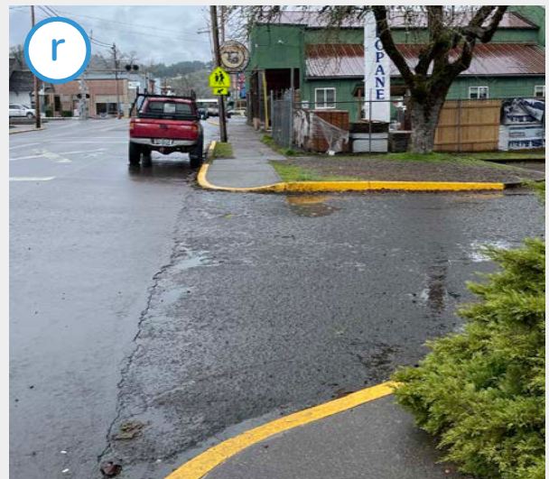
Yellow-painted curbs are intended to prevent parked cars from blocking the visibility of pedestrians crossing the street, but are sometimes disregarded in the absence of proper signage to reinforce them.
