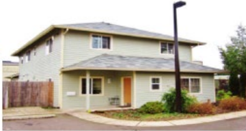
Mill Creek, Men's Home
